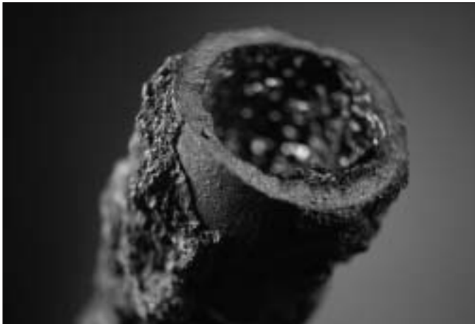
Some biofilms cause serious problems when they establish colonies inside metal piping and hasten corrosion.
